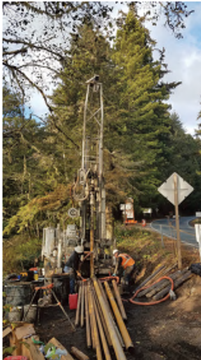
CME-850 track rig adjacent to southbound Highway 101. RC-20-013 (VWP-6) Gregg Drilling
