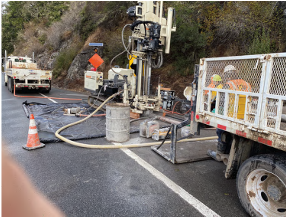
Geoprobe 3230 air rotary rig on northbound shoulder of Highway 101. P-20-012 (VWP-2SP) Gregg Drilling
