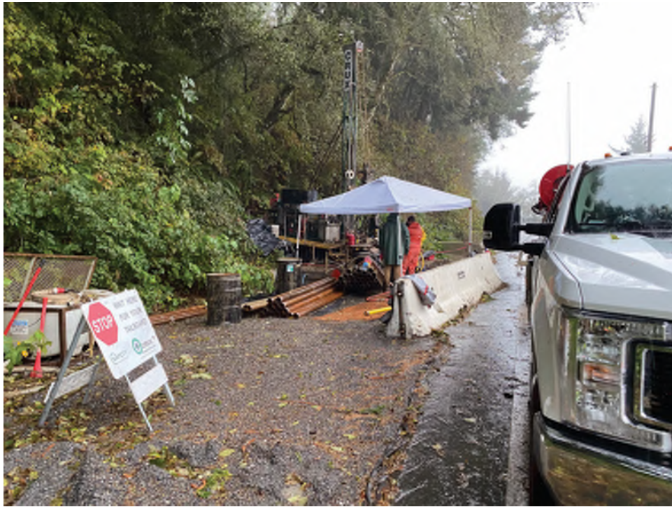
Burley 55-1 track rig adjacent to northbound shoulder of Highway 101. RC-20-016 (VWP-3) Crux Subsurface
