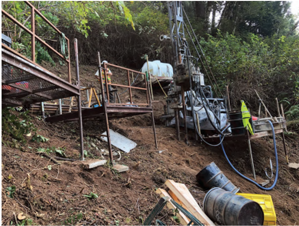
Burley 6000 helicopter access rig in State park. RC-20-005 (B-28) Crux Subsurface
