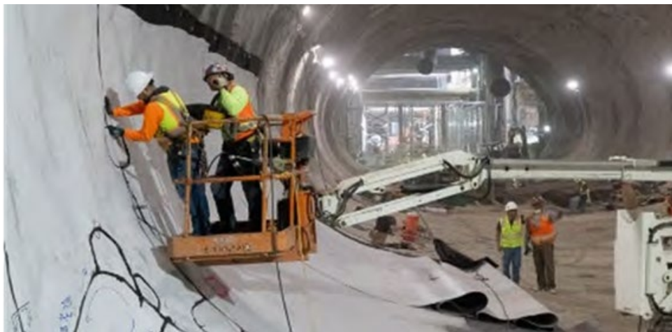
Figure 6. Membrane Waterproofing
