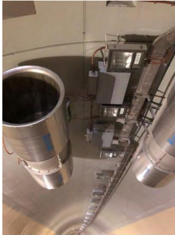
Figure 15. Jet Fans with In-tunnel Controllers (shown without screens)
