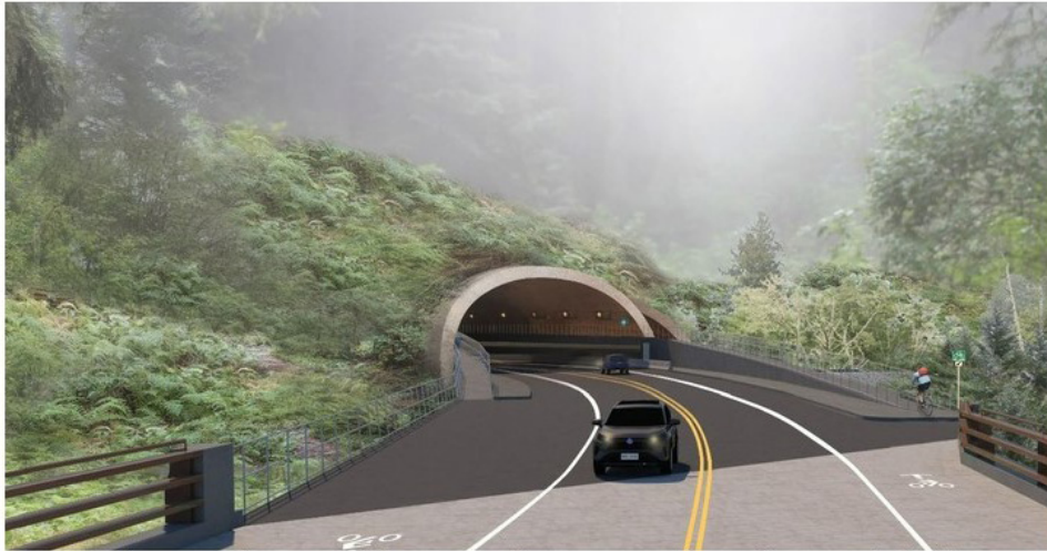
Alternative F, one of two potential permanent bypasses around Last Chance Grade, involves a 6,000 foot tunnel and includes a $1.4 billion price tag. | Image courtesy of Caltrans District 1
