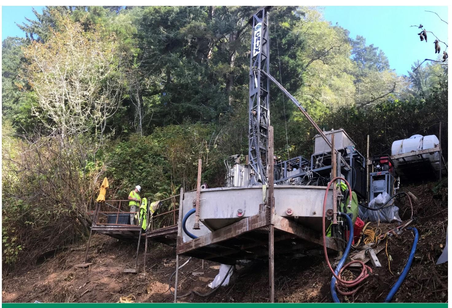
While Caltrans has completed geotechnical borings in the area to learn more about the landslides, both Alternatives X and F require additional geotechnical investigation. The photo shows an example of drilling equipment used, set on a platform that helps keep impacts minimal.
