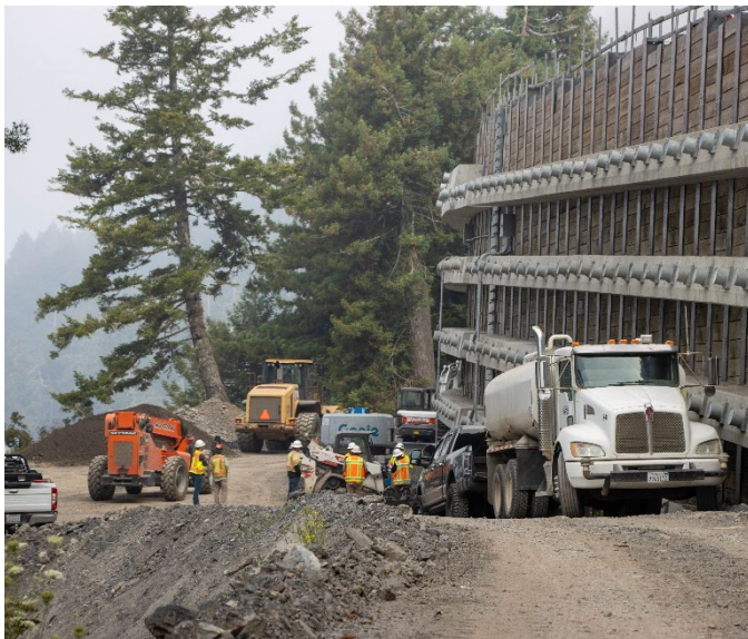
Finalizing construction of Retaining Wall No.5B at Last Chance Grade
