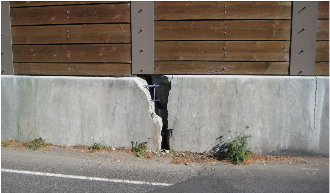
Figure 3 Cracking on Retaining Wall at NLCG and SLCG Slide Interface Near PM 15.2
