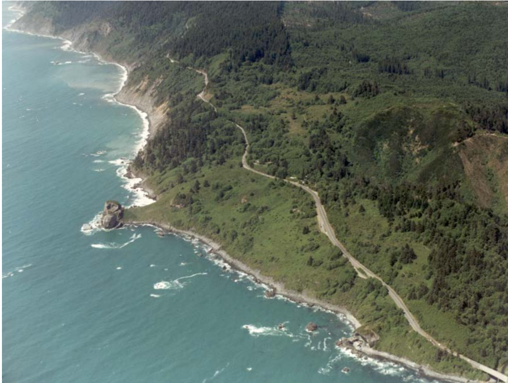
Figure 2. View north over Last Chance Grade area. From the Wilson Creek Bridge at lower right, Highway 101 crosses an earthflow complex above Footsteps Rock (left center), then crosses into much more resistant bedrock characterized by deep-seated rock slides and surficial debris slides.
