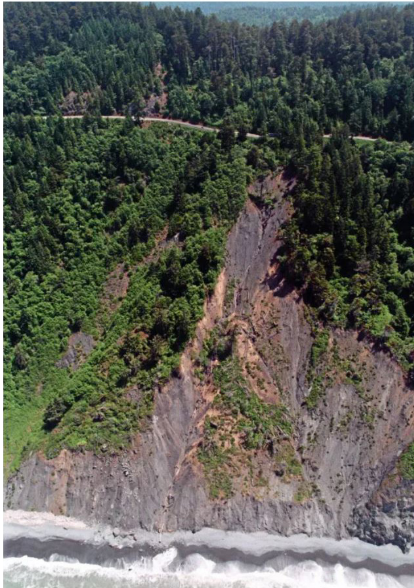
The Last Chance Grade section of Highway 101 about 10 miles south of Crescent City has experienced over 200 landslides due to its unstable coastal geography. A new plan aims to improve it. – Photo courtesy of Tamera Leighton
