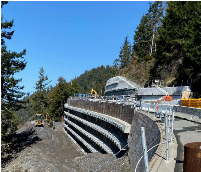
Current construction at Last Chance Grade (Retaining Wall No. 7)
