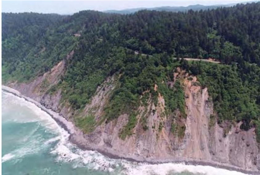
Last Chance Grade, an oft-closed and perilous section of Highway 101 just south of Crescent City. Photo: Caltrans.
