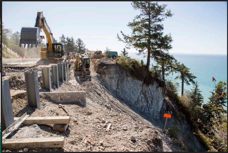
Wilson Creek Wall New Retaining Wall Southern End of Last Chance Grade
