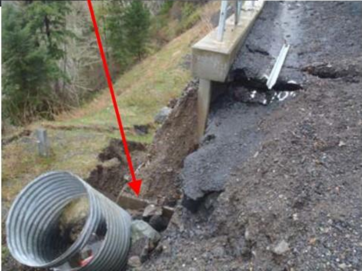
Failing Wall Lagging / Failing Barrier / Failing Shoulder & DI
